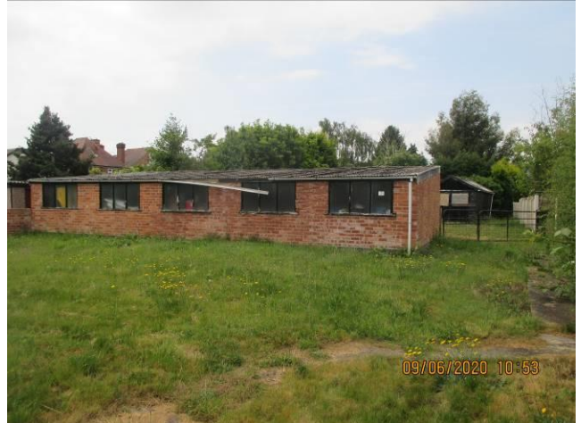
View of garages facing west
