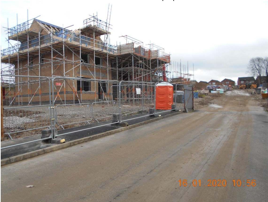
View of north side of Alton Drive towards rear of properties on Robina Drive.
