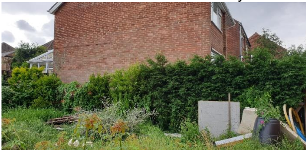
Side elevation and rear of 11 Kirby Close
